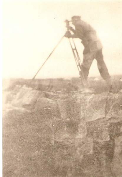
Figure 11 Survey at work 2
