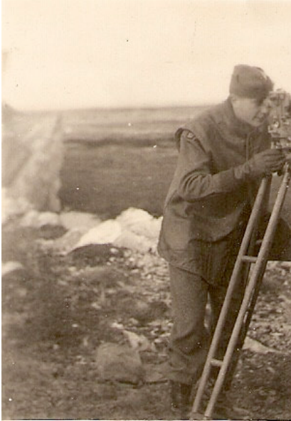
Figure 10 Survey at work 1
