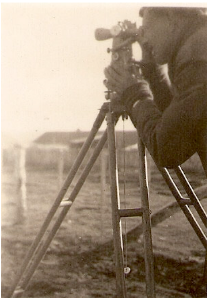
Figure 12 Survey at work 3
