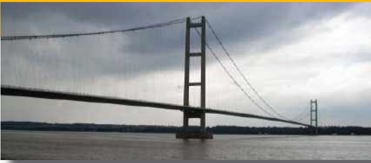
The Humber Bridge – a recent survey task for KJ Hall Surveyors – including Ken.
