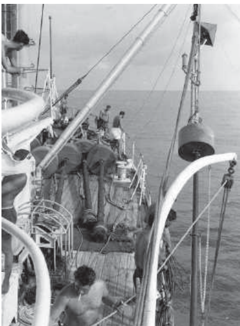
HMS Dalrymple beacon laying
