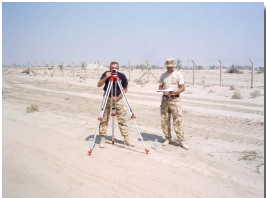
Check levelling the Shaibah Logistics Base access road.
