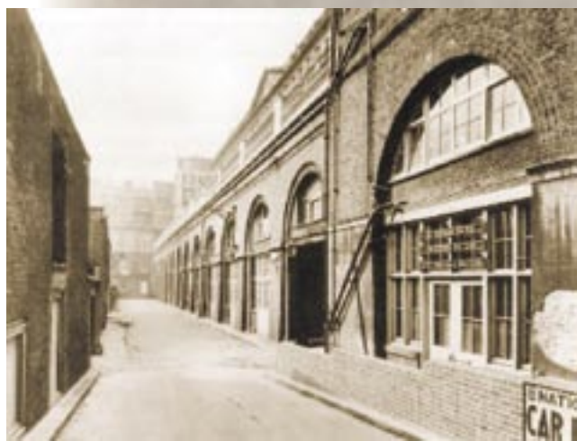
Adelphi Terrace, Whitehall. Converted coach house and stables which served as the first home of the Topographical and Statistical Department of the War Office (1855-56)
